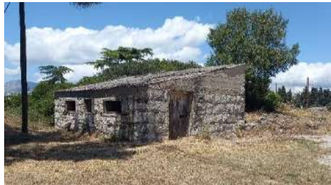
Figure 28. Auxiliary building 1 (Storage – cadastral parcel no. 7372) for storing tools, etc.
