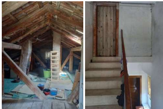
Figure 22. The attic of the Building 2A
