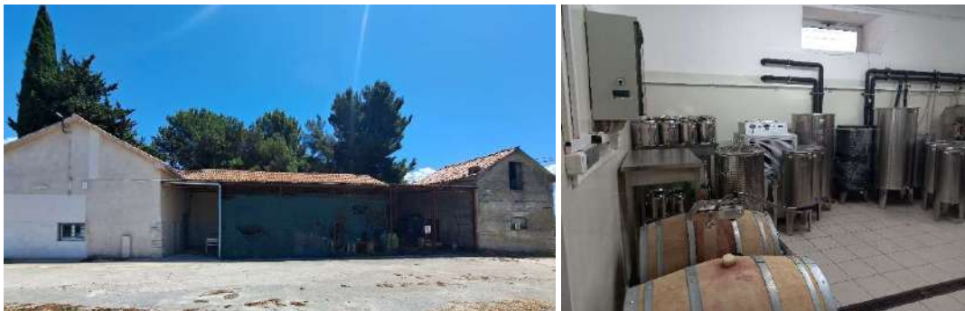
Figure 29. Auxiliary building 2 (Storage – cadastral parcel no. 7391; experimental wine cellar)
