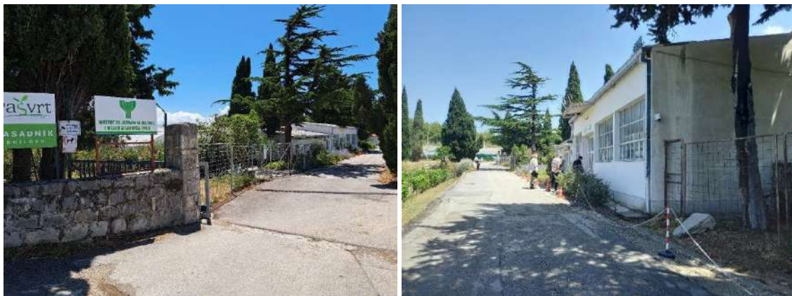
Figure 8. The existing Building A planned for reconstruction
