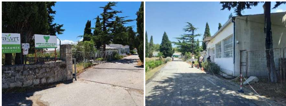
Figure 8. The existing Building A planned for reconstruction
