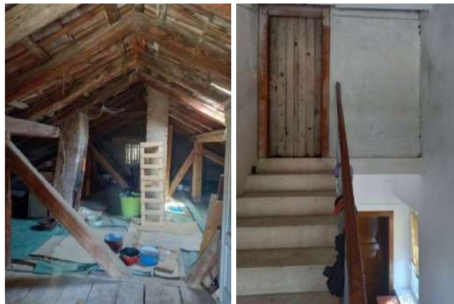
Figure 22. The attic of the Building 2A
