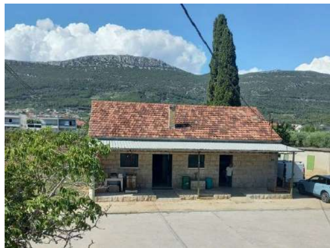
Figure 23. The existing Building 2B (experimental oil mill) planned for improvement
