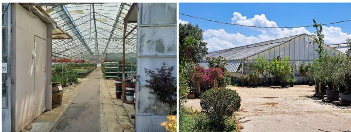
Figure 9. The existing Building B (greenhouse) planned for reconstruction
